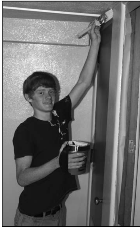
Shawn Barron paints in Fellowship Hall. Shawn coordinated the Fellowship Hall painting as part of an Eagle Scout project.
