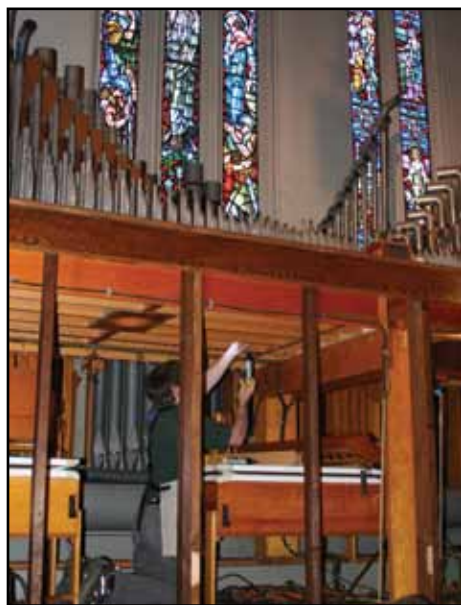
A worker removes the bottom boards connected to each pipe
